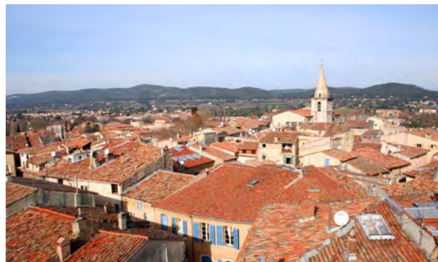
View of Brignoles - Photo : service de communication de Brignoles
